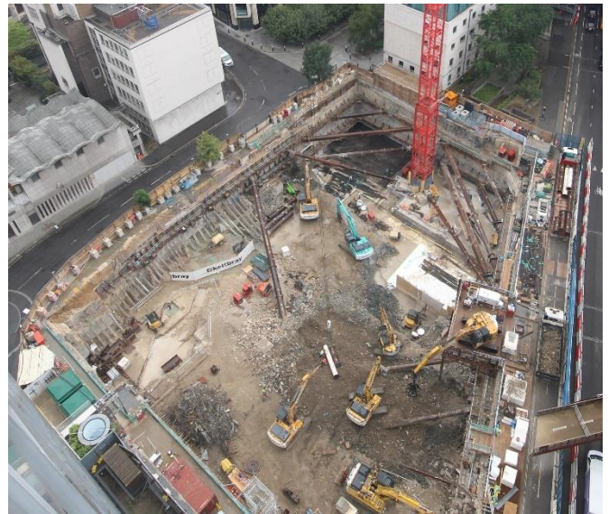
Overview of site progress
