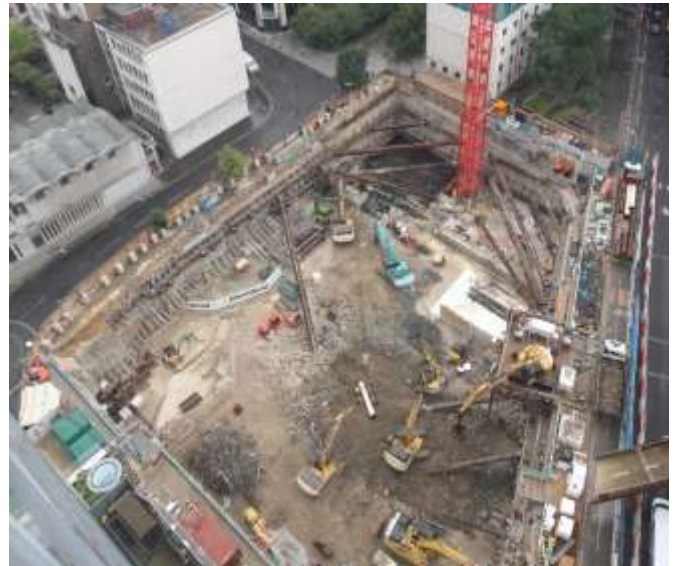
Overview of site progress
